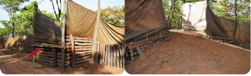
To eliminate the potential gap (see red arrow above) between the truck opening and the offloading ramp, an extra pole or piece of conveyor belt may be used.
